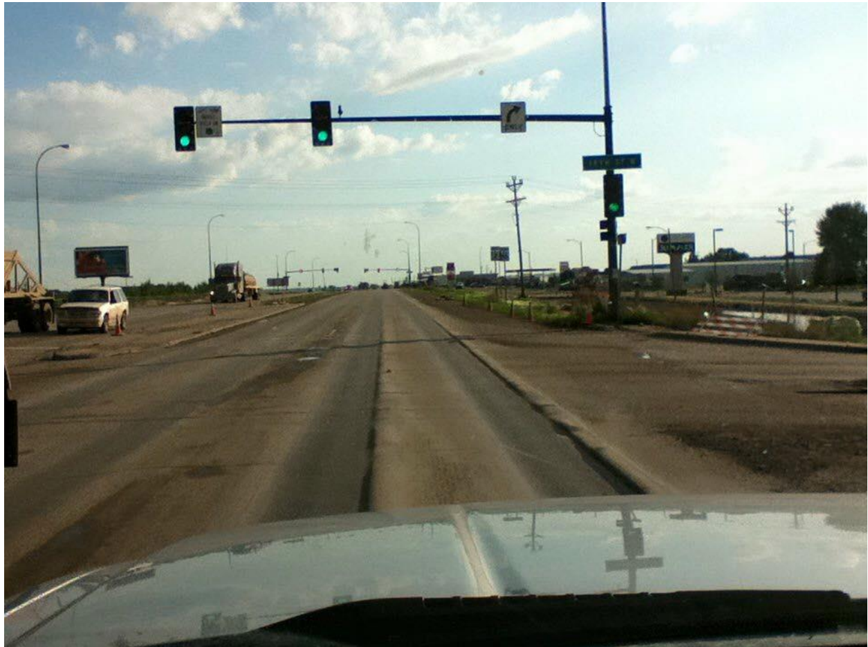
Figure 16. Photograph of ruts created in the streets of Williston, North Dakota by oil trucks and increased traffic in 2010. Taken from “Bakken Oilfield Fail of the Day” Facebook posted May 15, 2016.
